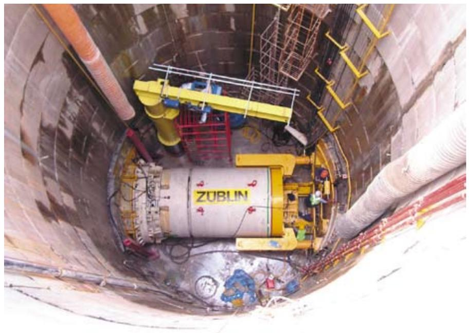
Pipe jacking from within the temporary shaft.
