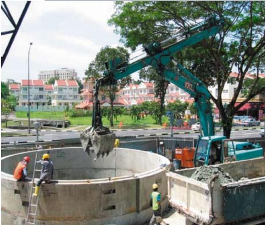
The caisson sinking method was used to construct the temporary shafts.
